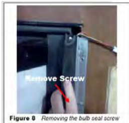
Figure 8 Removing the bulb seal screw
